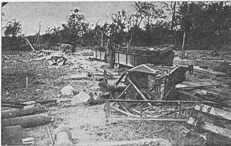
8. Breech end of wrecked ramp at Site No. 18. The end of this ramp shows the interrupted flange to which the combustion chamber is attached.
